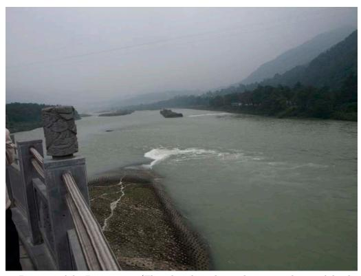
Photo 4 Damage of the Dujiangyan (The white line shows the repaired part of the damage  $\,$  )
