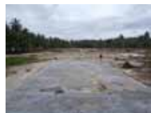
Damage in Muntei
