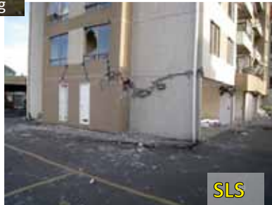
Salas 1343 building Heavily damaged building at Concepción city during the 2010 Maule earthquake
