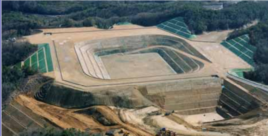
Construction Site (January, 2000)
