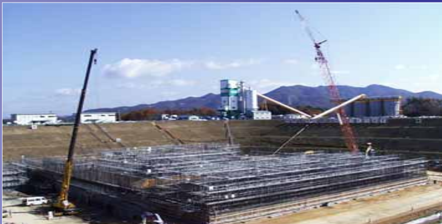
Experiment Building Foundation (April, 2001)
