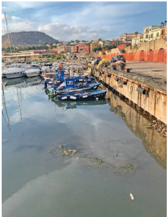
Pozzuoli, a port town in the Campi Flegrei volcanic area, Italy. Uplift of the ground has created a visible gap between the quay and the sea level.
