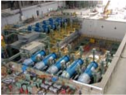
Figure 8: Installation of H-Actuator
