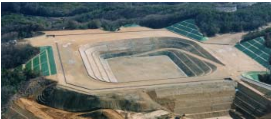
Figure 3: Construction Site (January 17, 2000)
