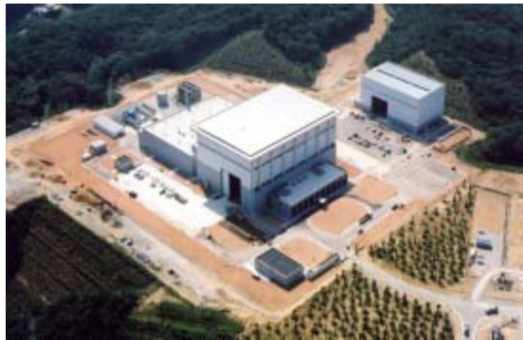
Figure 5: Recent Construction Condition
