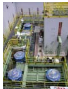
Figure 7: Installation of V-Actuators
