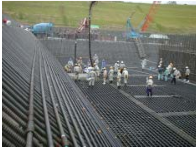
Figure 4: First Concrete Casting (June 20, 2000)
