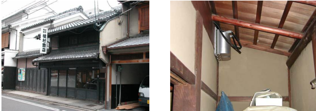
Photo 4 Wooden house and installed observation seismograph
