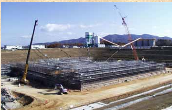
Experiment Building Foundation (April, 2001)
