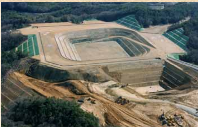
Construction Site (January, 2000)
