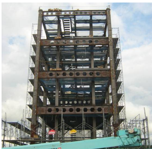
(a)鉄骨の建て方
