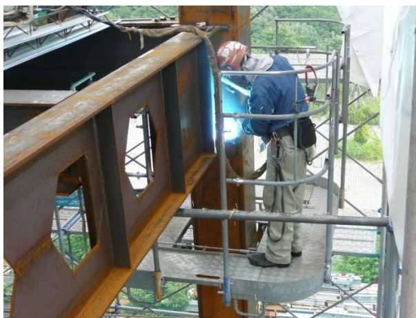
(b)梁の根元の現場溶接
